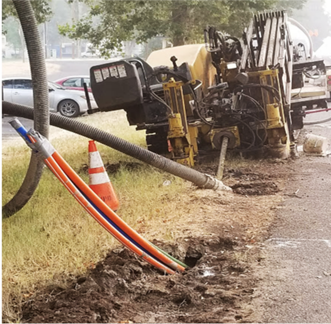
Figure 3-7: Horizontal Drilling Rig and Conduit
